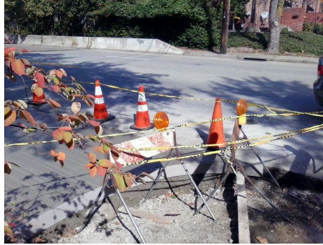
Figure 7.1 A wooden spline used to create a smooth, curved border for a paved area (Shadyside, Pittsburgh, October 2014).
