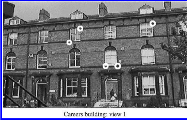
Figure 23.2 One view of the Careers Buildings (University of Leeds) with five landmarks.
